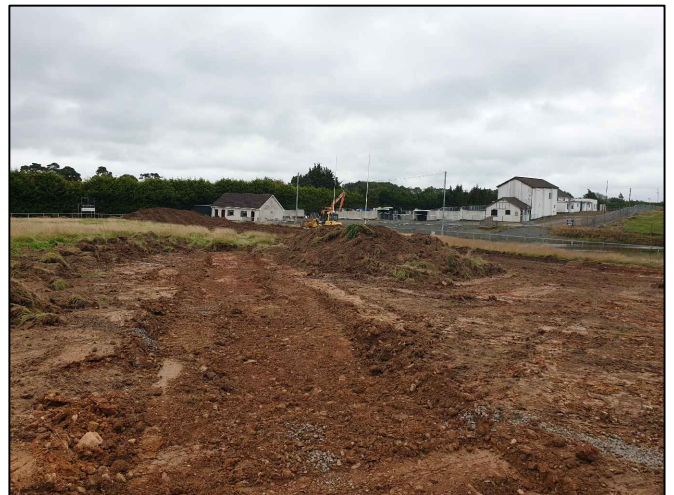
Plates 3 and 4: Stripping of Vegetation and Topsoil (August 2019)
