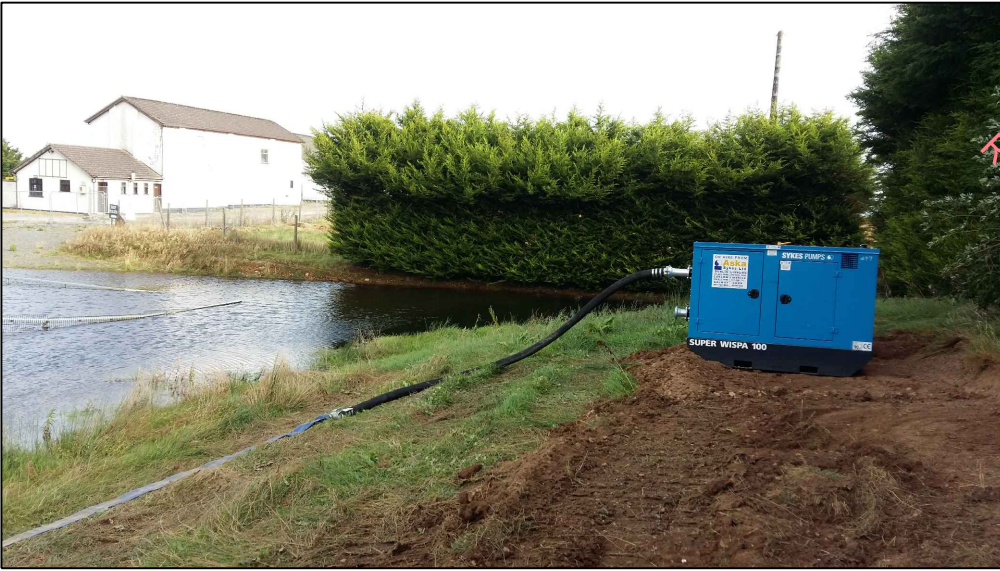
Plates 5 and 6: Pumping and discharging ponded water (Sept 2019)
