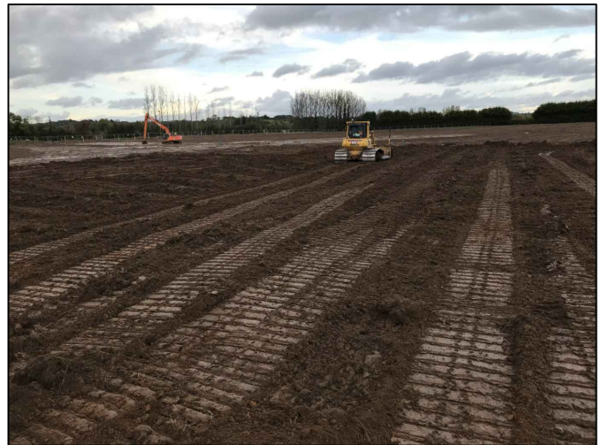
Plate 26: Spreading Topsoil
