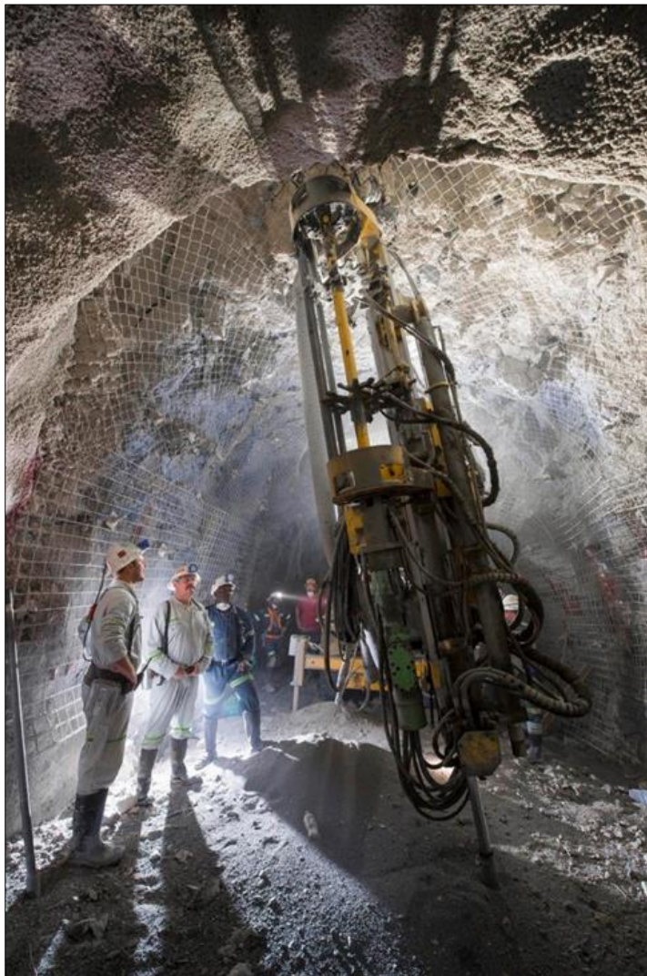
Figure 6: Rock bolt and mesh installation
