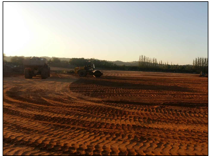
Plates 17 and 18: Re-profiling and grading (Sept 2019)
