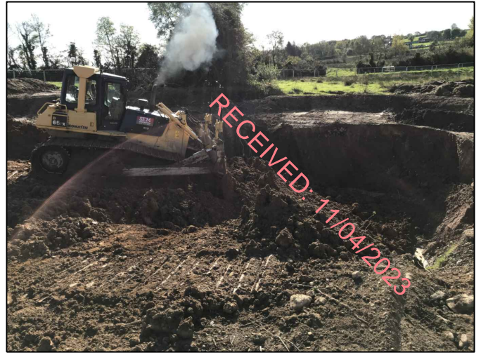
Plates 27 and 28: Infilling Crown Hole (21 Oct 2019)
