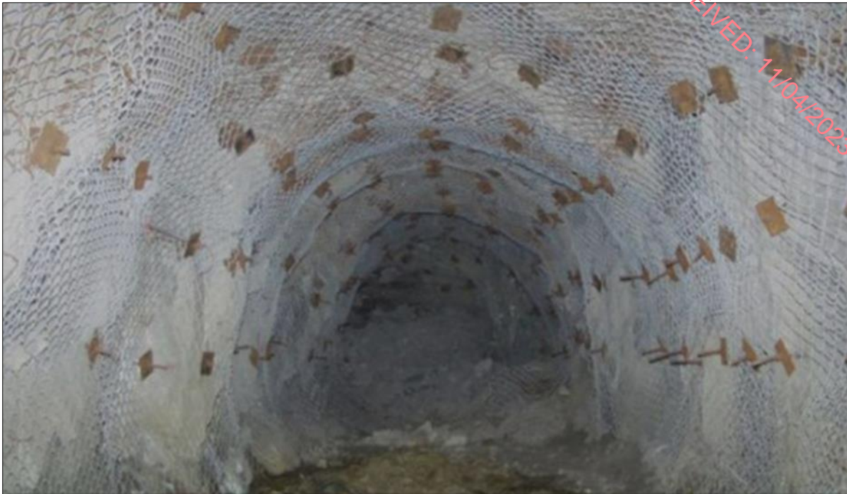
Figure 7: Example of installed rock bolt and mesh
