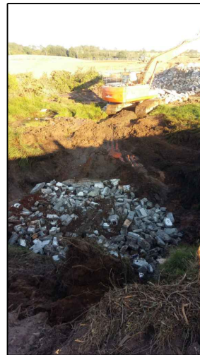
Plates 19 and 20: Pumping down Crown Holes and Infilling (Sept 2019)
