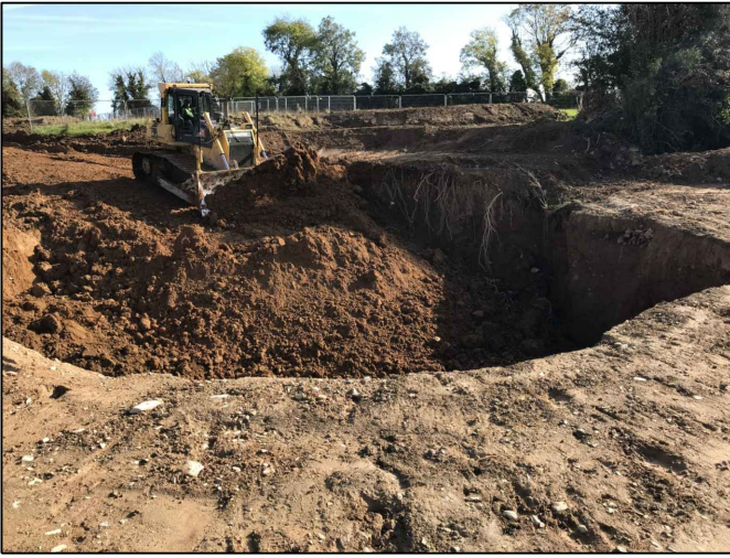
Plates 27 and 28: Infilling Crown Hole (21 Oct 2019)
