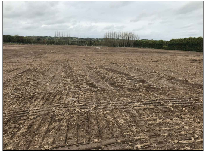
Plates 29 and 30: Grading and sealing surface prior to hiatus (23 Oct 2019)
