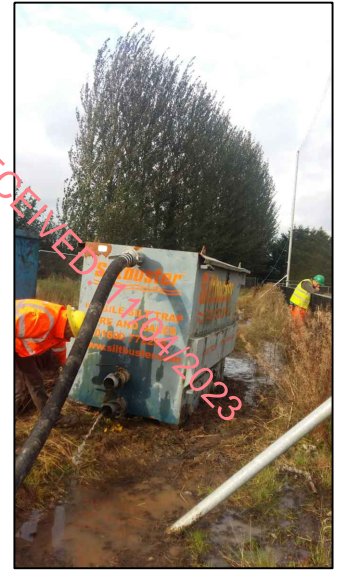
Plates 5 and 6: Pumping and discharging ponded water (Sept 2019)
