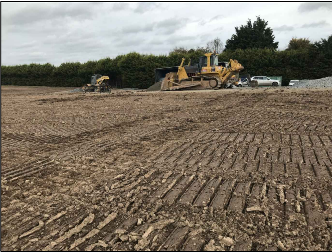
Plates 29 and 30: Grading and sealing surface prior to hiatus (23 Oct 2019)
