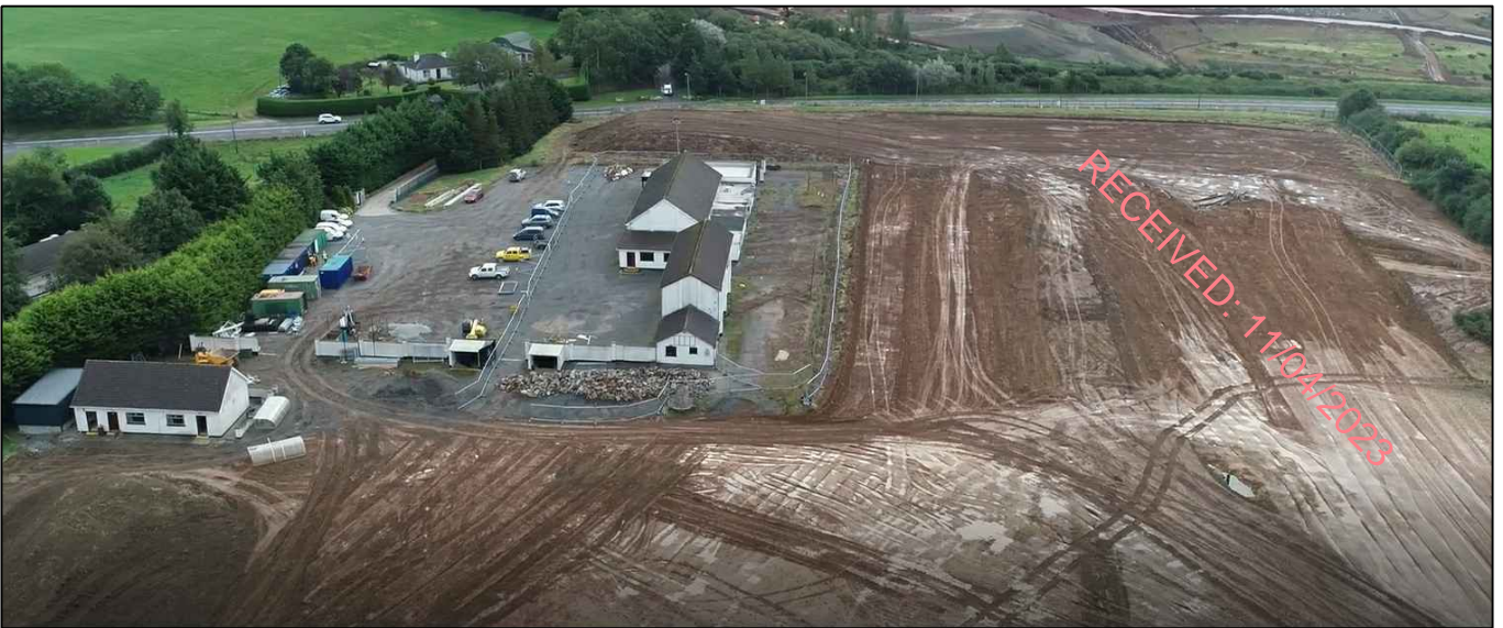
Plate 11: Project Progress - Extent of Soil Stripping (11 Sept 2019)
