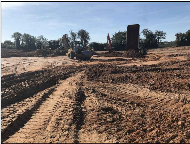
Plates 17 and 18: Re-profiling and grading (Sept 2019)
