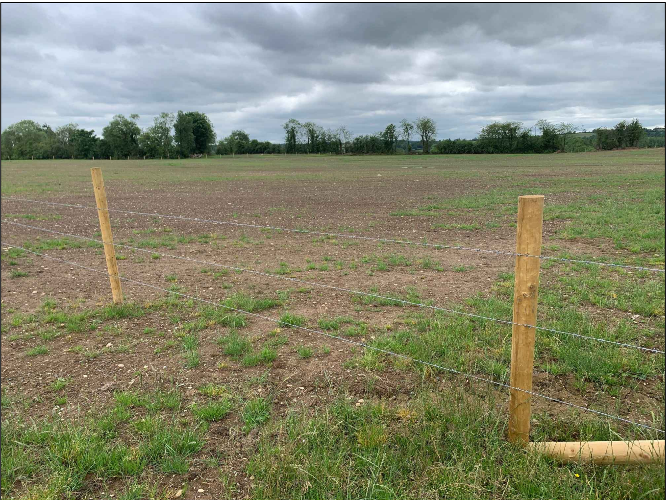
Plate 41: Completed Works (July 2020)
